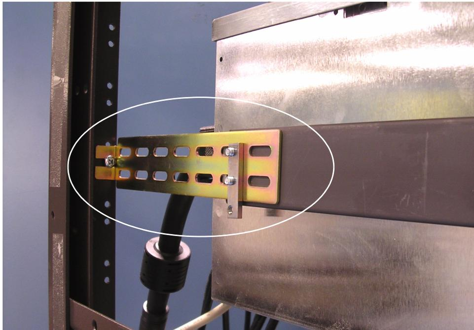
Figure 3-2. Extra brace added to rack slide.
