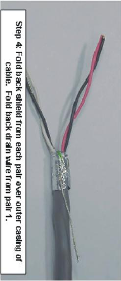
Step 4: Fold back shield from each pair over outer casing of cable. Fold back drain wire from pair 1.
