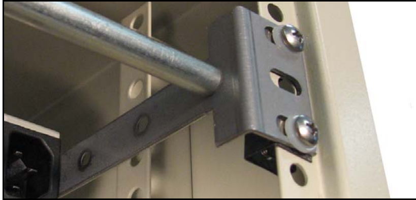
Figure 2-5 Installed Support Arms and Cable Relief Bar
