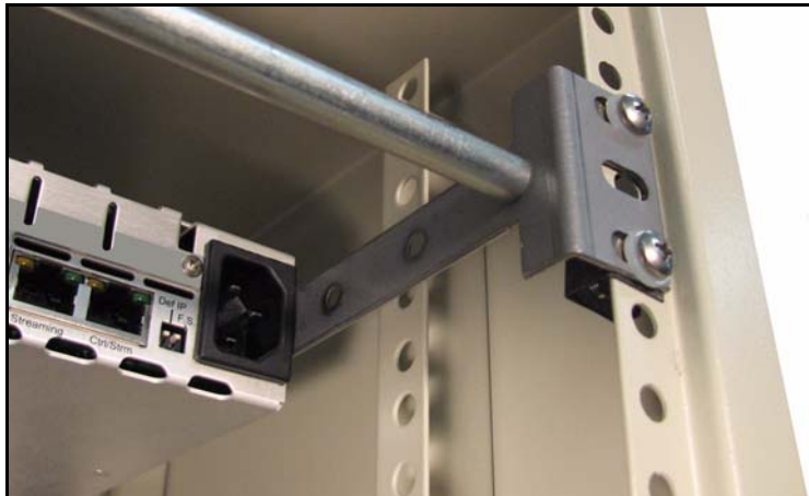
Figure 4-4. Installed Support Arms
