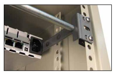
Figure 4-4. Installed Support Arms
